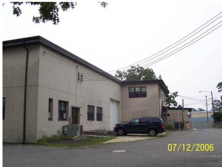
Fort Monmouth, Building 292, Museum Storage (West)
