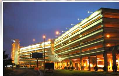
Philadelphia International Airport Parking Garage Philadelphia, PA
