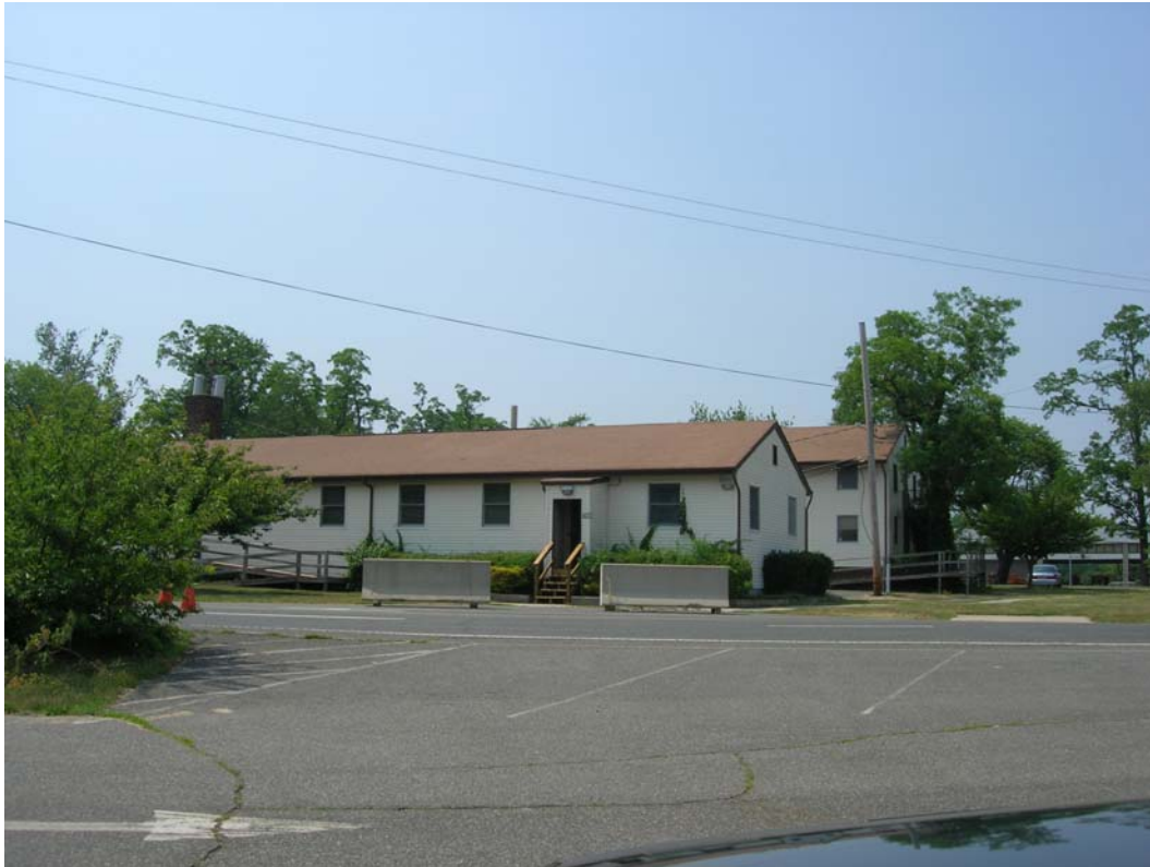
Figure 7-25: Typical one-story temporary structure rehabilitated for office space, with a two-story unit beyond.
