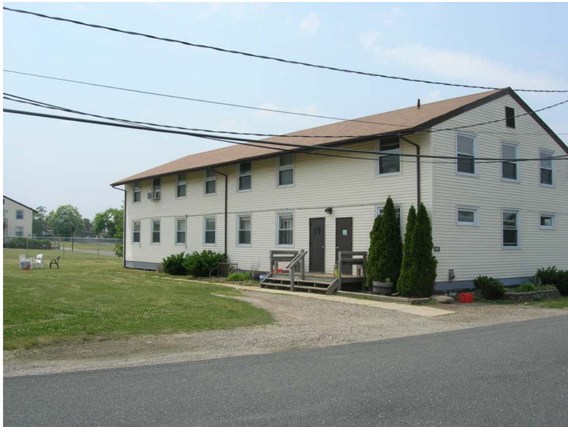
Figure 7-9: Temporary wood structure (Photo courtesy of FMERPA)
