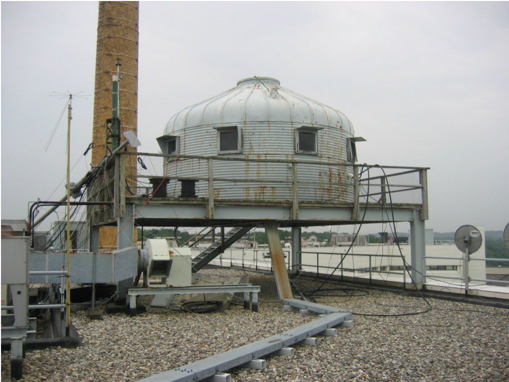
Figure 7-23: The Dymaxion Deployment Unit should be placed on a concrete foundation, and all materials restored to their original condition.
