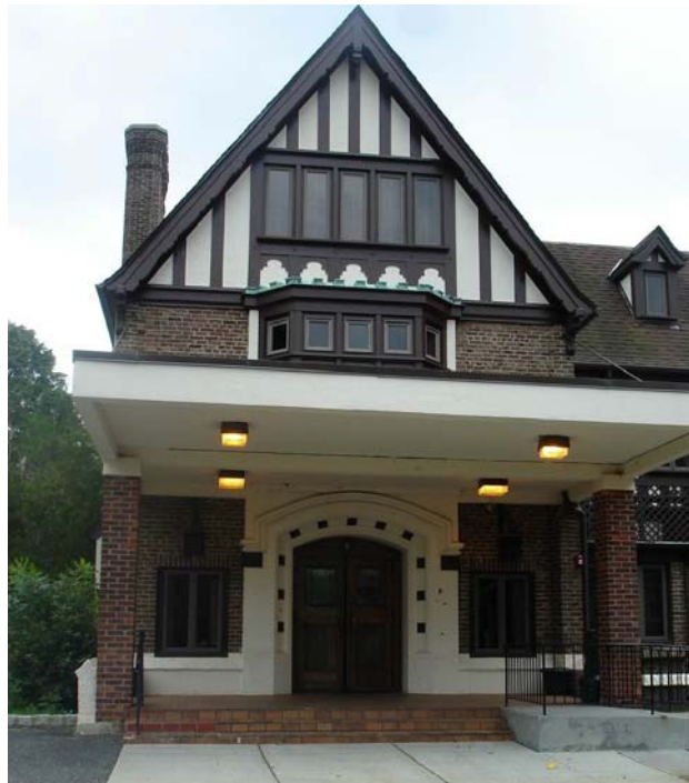
Figure 7-19: The sheltered entrance to Gibbs Hall is appropriate for a golf clubhouse or hospitality center.
