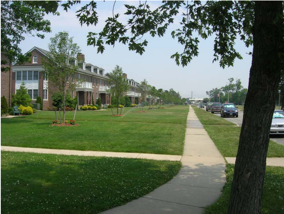
Figure 7-12: Family housing surrounds the Parade Ground at the north and south. (Photo courtesy of FMERPA)
