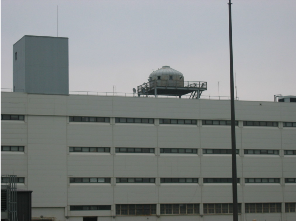
Figure 7-10: Dymaxion Deployment Unit at roof as seen from the ground.
