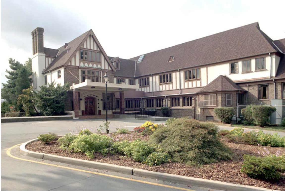
Figure 7-2: Gibbs Hall serves as a dining facility and club house for the Suneagles Golf Course (Photo courtesy of FMERPA)
