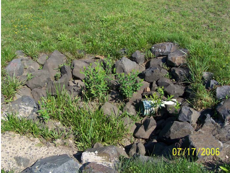
Fort Monmouth, Building 2560, Discharge from Water/Oil Separator
