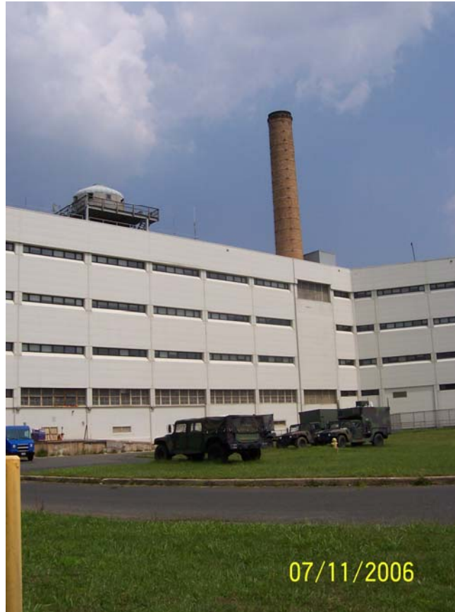
Fort Monmouth, Building 2700 – Myers Center, Paper Waste Incinerator and Boiler Stack
