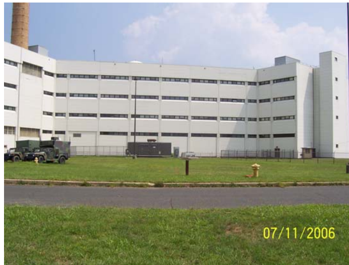
Fort Monmouth, Building 2700 – Myers Center
