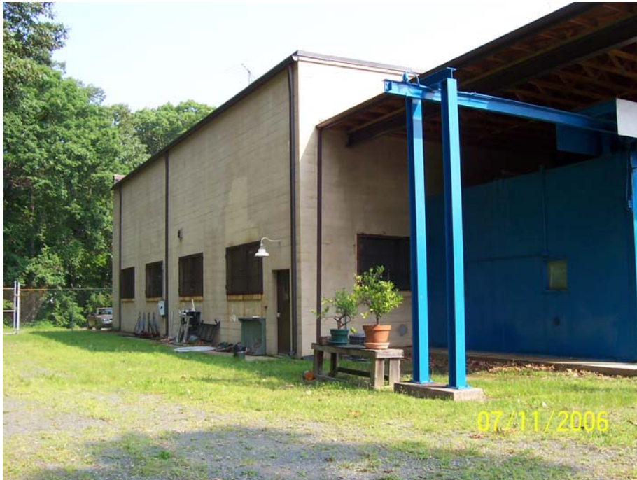
Fort Monmouth, Building 2704 (West)
