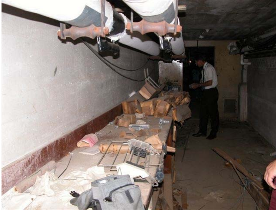
Fort Monmouth, Building 283 – Squier Hall, Basement Workroom
