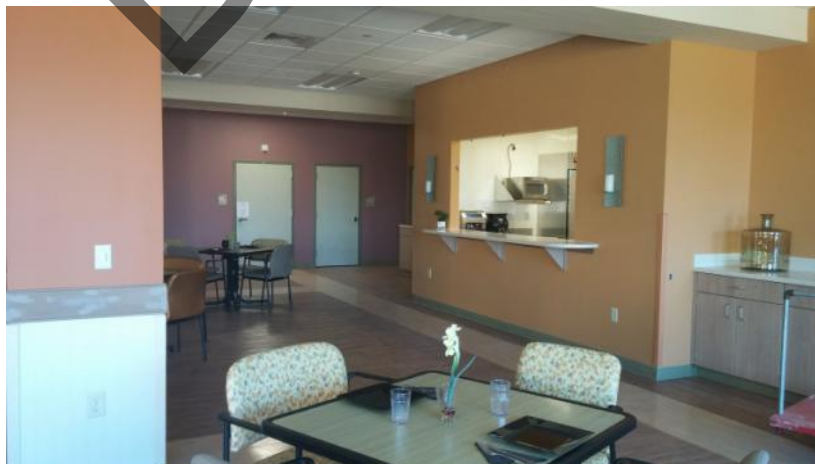
Interior renovations at the former Patterson Army Clinic
