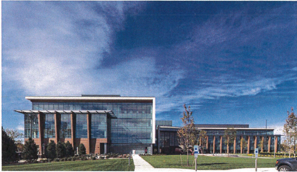
Commvault's world headquarters, located at Fort Monmouth in Tinton Falls. Commvault was honored with a Leading Economic Development/Redevelopment Award for its role in revitalizing the region
