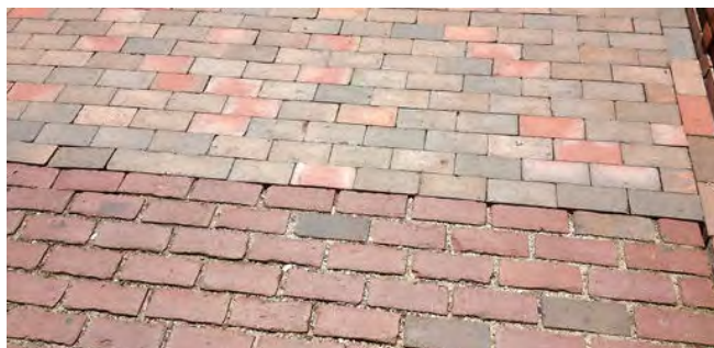
Top left: Inappropriate mortar, size, texture and color
