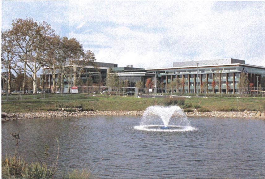
CommVault's new Headquarters located across Hope Road from Howard Commons
