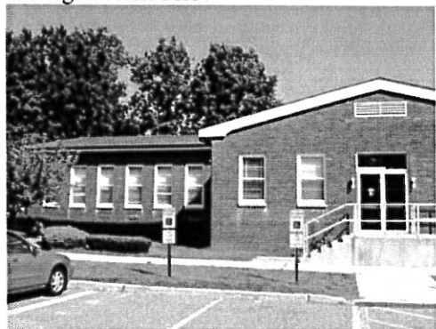
Side entrance to addition
