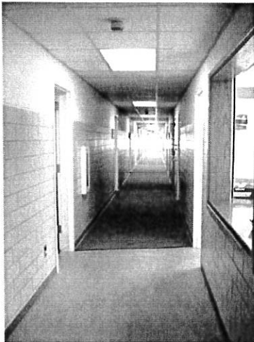
View of classroom corridor
