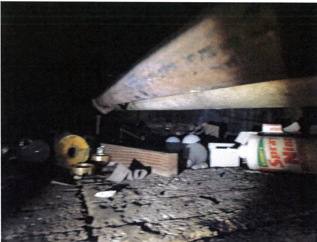
Basement, Room B-12A: Damaged pipe insulation and debris above freezer.
