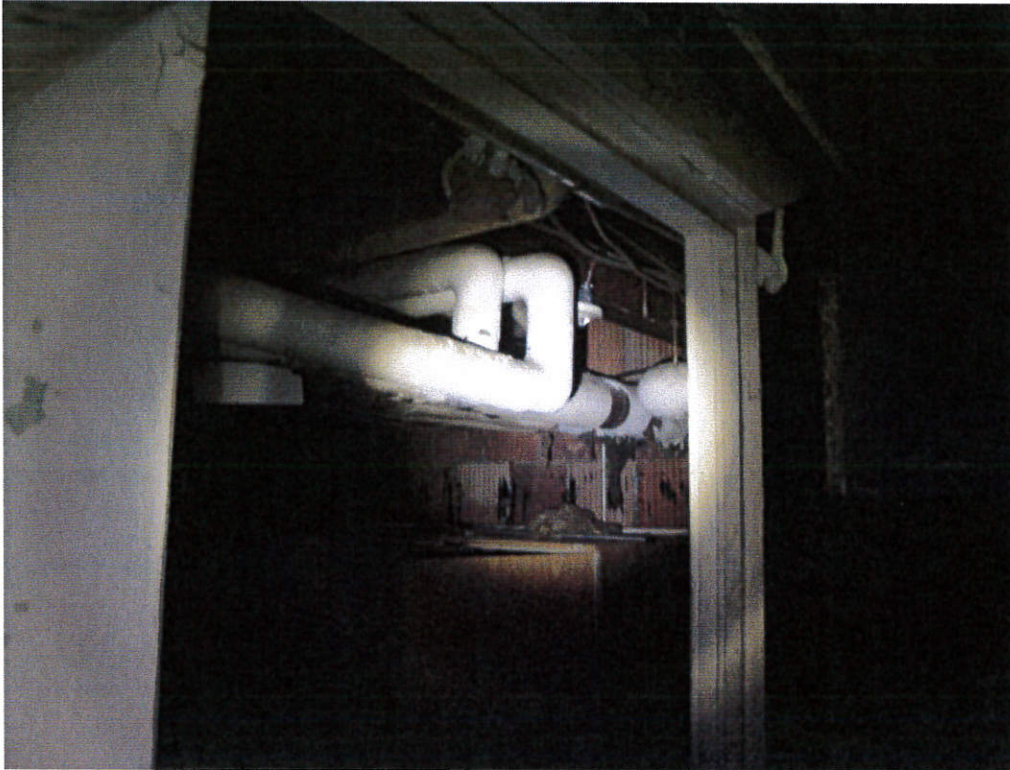
Basement, mechanical room (north): Damaged pipe insulation.
