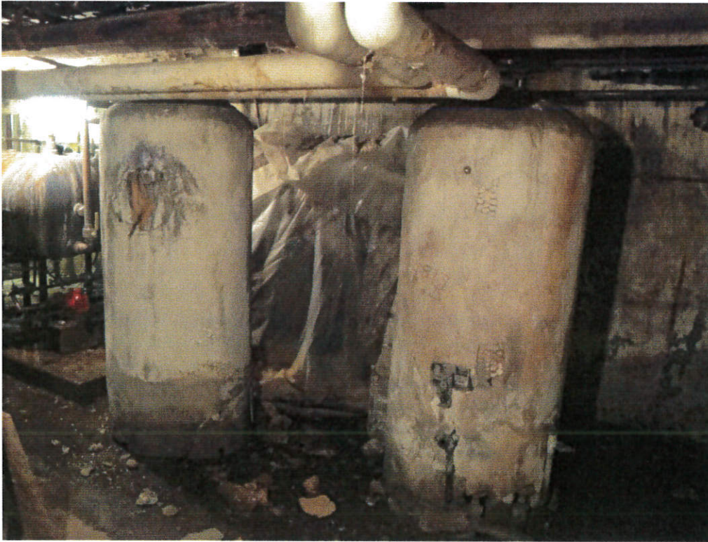
Sub-basement, Boiler Room B-1: Damaged tank insulation.
