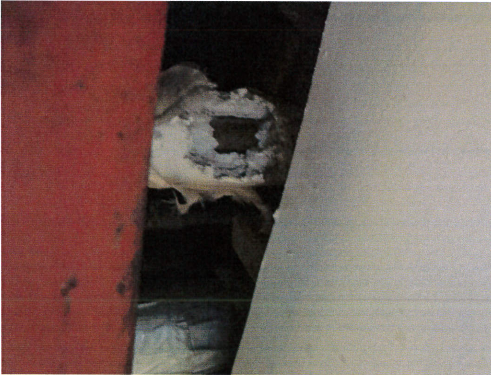
Basement, mechanical room (south): Damaged ACM pipe fitting.
