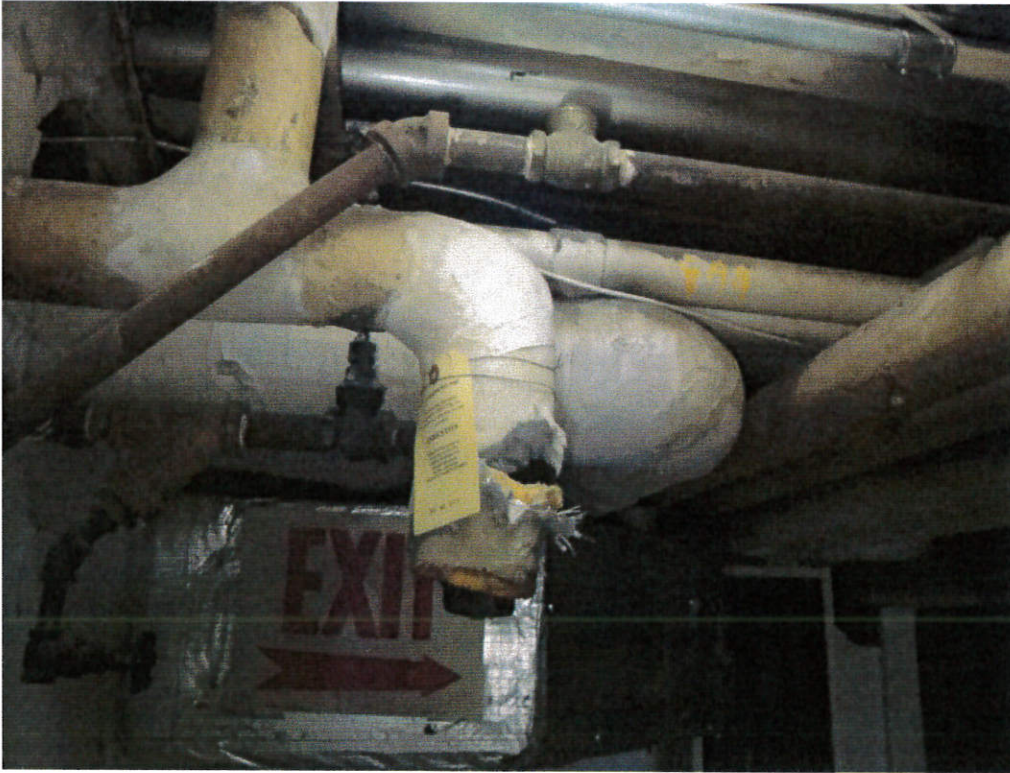
Basement, Corridor B: Damaged pipe fitting.
