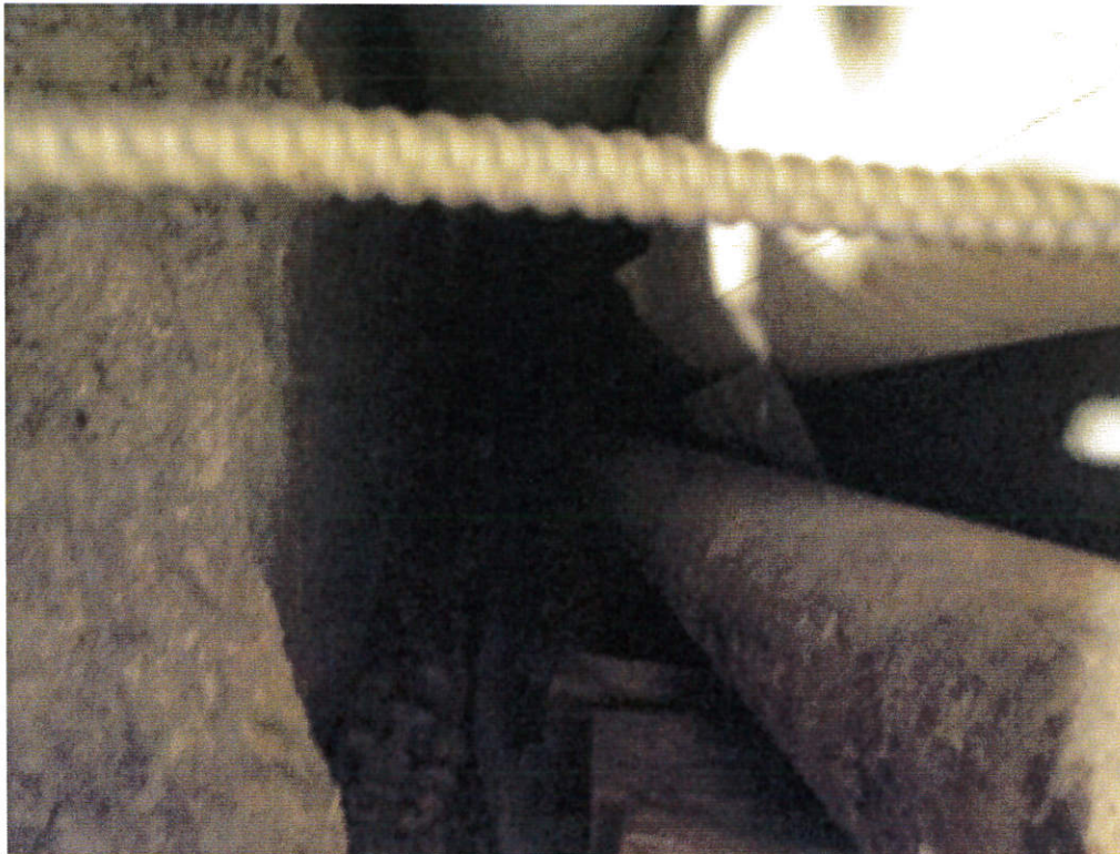
Sub-basement, Boiler Room B-1, pipe tunnel: Damaged pipe insulation and debris.
