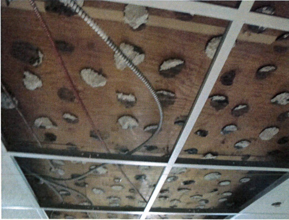
Building 2000, basement, bar area: Suspect ceiling tile glue.
