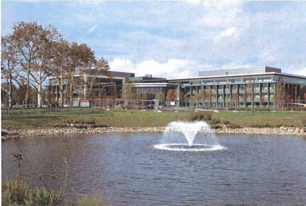
CommVault's new headquarters located in the Tinton Falls section of Fort Monmouth
