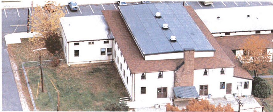
View of Building 552, the former recreation center, from Brewer Avenue
