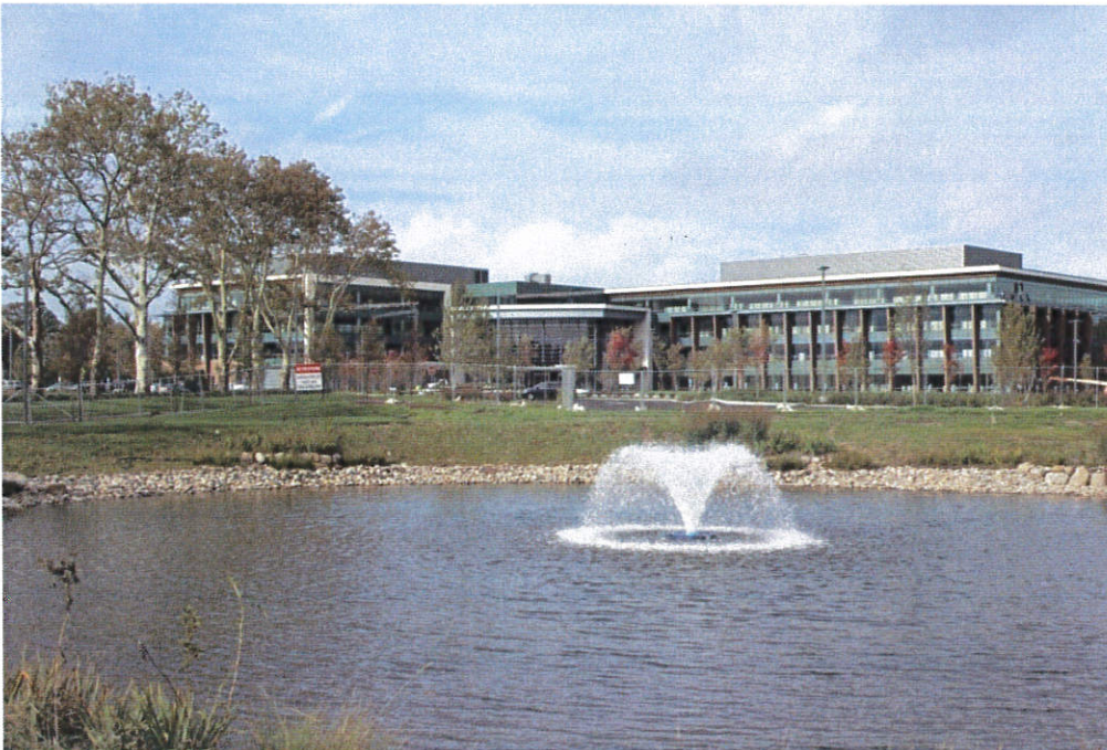
CommVault’s new headquarters located in the Tinton Falls Reuse Area
