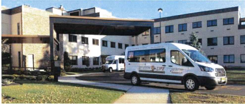
AcuteCare's renovated facility, located in the Oceanport Reuse Area
