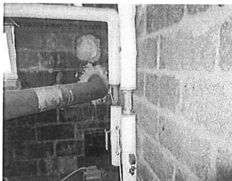
Typical new fiberglass pipe insulation in the basement.
