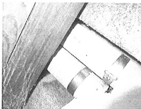
PACM visible going behind the wall on Second Floor risers.
