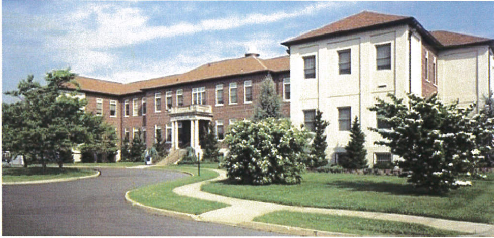
Historic Allison Hall, Building 209
