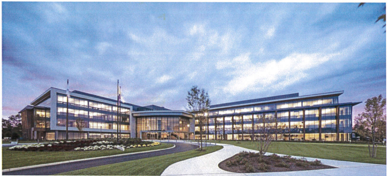
Commvault's new Headquarters on Fort Monmouth
