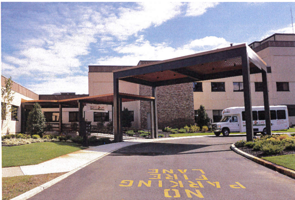
AcuteCare's renovated facility
