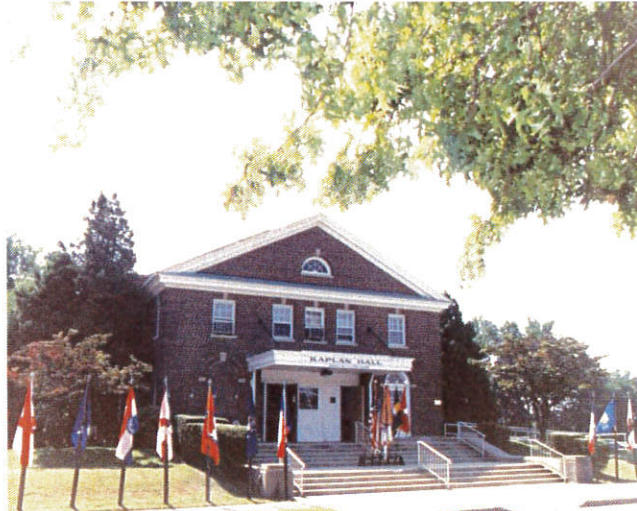
Kaplan Hall, Building 275
