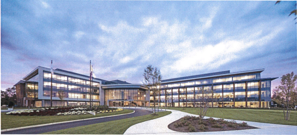
CommVault's new Headquarters
