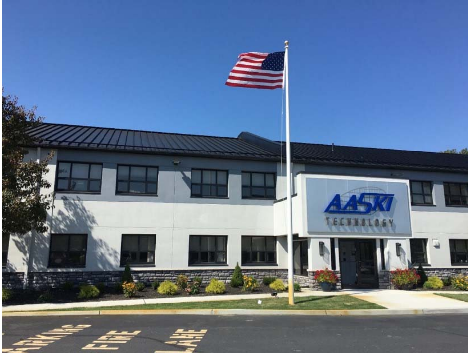
Building 2525 in Tinton Falls, home of Aaski Technology
