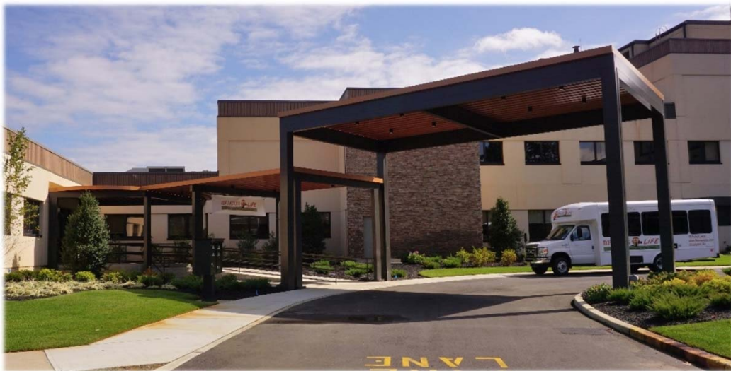
AcuteCare's renovated facility in the Oceanport Reuse Area
