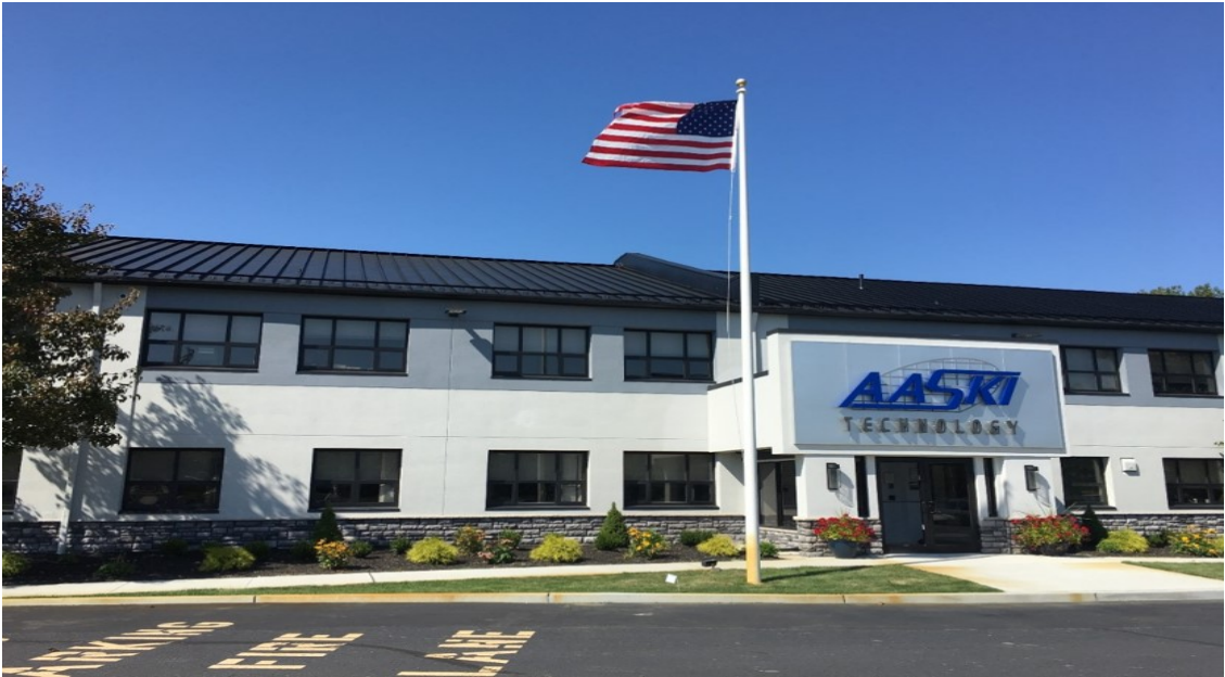
Building 2525 in Tinton Falls, home of Aaski Technology
