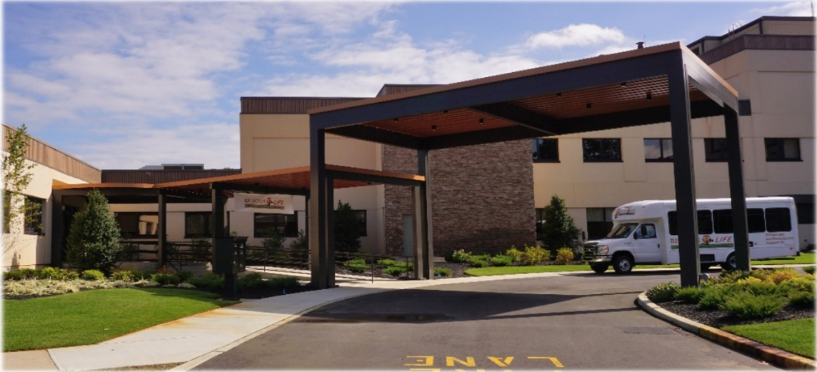
AcuteCare’s renovated facility in the Oceanport Reuse Area
